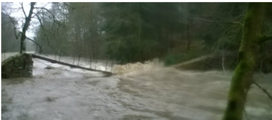
Allen banks bridge damaged in the flooding
