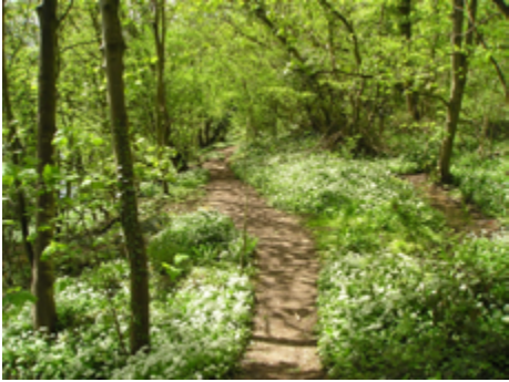
Re-surfacing work in Darlington Borough on the Teesdale Way
